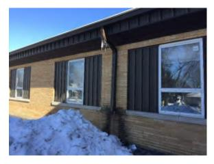
Photo 25. Windows at 1954 original building. Thermal imaging showed no major temperature issues here.
