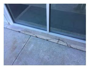
Photo 30. Concrete cracking at top of concrete foundation wall. Joint should be caulked to avoid future freeze/thaw concern. (Priority 0)
