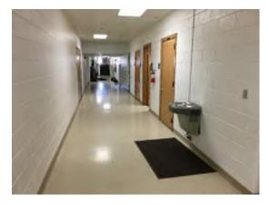
Photo 47. VCT flooring at 1954 building corridor. Lower level shown here in fair condition. At upper area to the east, flooring in poor condition and should be replaced.
