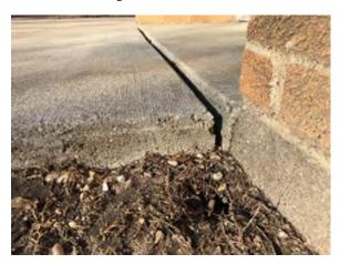
Photo 2. Sidewall is pulling away from the stoop slab. Slab should be tie in to the stoop wall to avoid differential movement. (Priority 2)
