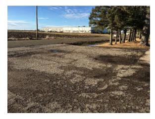
Photo 5. Asphalt in poor condition with cracking and potholes throughout. Replace and restripe. (Priority 0).
