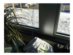
Photo 18. Solid surface window sills at south elevation of 1963 original classrooms are in good condition.
