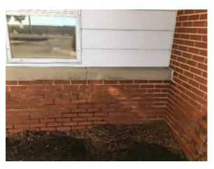
Photo 14. Mortar cracking and discoloration. Typical on west
