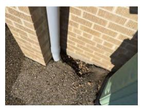
Photo 5. Patch to minimize potential for water infiltration below grade. (Priority 0)
