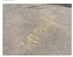
Photo 4. Parking striping fading. Consider restriping parking lines and other markings.
