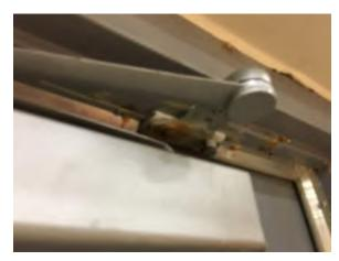
Photo 27. Door frames on the north elevation of the 2001 gymnasium are showing significant amount of surface rust. District will remove and repaint.
