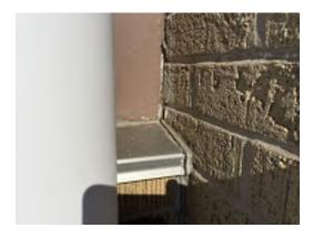
Photo 3. Detail at window and adjacent wall on building south elevation. Review caulking and sealing when differing materials intersect. (Priority 0)
