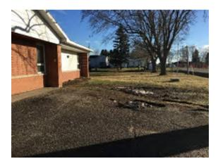
Photo 9. Asphalt in poor condition with cracking and potholes throughout. Replace and restripe. (Priority 0).
