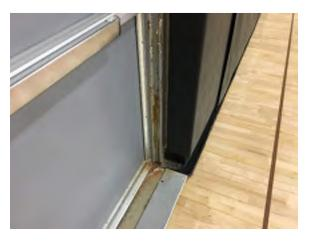
Photo 31. Door Frames along north end of Gymnasium (2001 Addition) show signs of surface rust. Prep and repaint to address.
