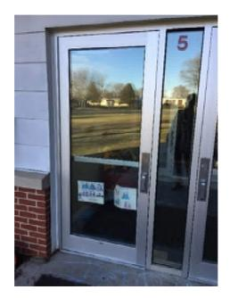
Photo 33. Exterior doors in at 2000 addition are in good condition.
