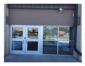
Photo 31. Entry on west side of north elevation in 1963 building. Key fob access only during the school day. Aluminum framing is failing at bottom of door jamb. (Priority 2)
