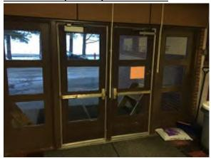
Photo 11. Interior of main entrance. Door electrification surface mounted.
