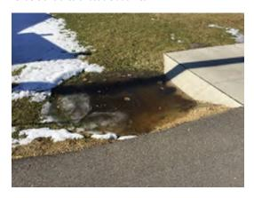
Photo 2. Storm inlet to the west of the baseball field plugged and not draining properly.
