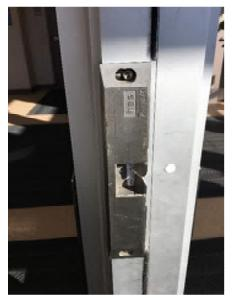
Photo 16. Electric strike at interior vestibule doors of 2012 addition main entrance. This secures interior set of doors and requires passage through main office to gain access to building.
