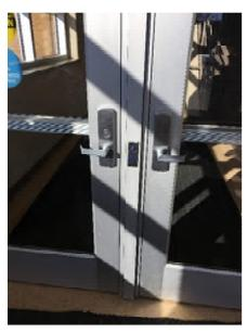
Photo 15. Main entry vestibule in 2012 addition. Doors have ADA auto opener button installed on mullion.
