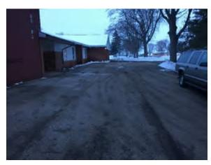
Photo 4. Asphalt in poor condition with cracking and potholes throughout. Replace and restripe. (Priority 0).
