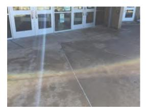
Photo 3. Concrete at HS main entry in good condition.
