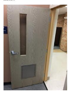
Photo 19. Wood door at conference room in 1999 addition. Door grille utilized for air transfer.
