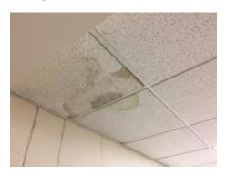
Photo 51. Stained ceiling tile at tie-in between 2001 addition (District Office Hallway) and 1963 original building. Install expansion control. (Priority 2)
