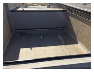
Photo 42. Roofing area enclosed on all four sides at 1963 building. Water sits in this location. There is ladder access to this area from the south.
