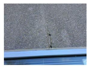
Photo 24. Crack is apparent in center of precast panel above window (same location as shown in photo 23)
