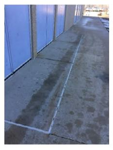
Photo 2. North exit doors from main Gymnasium. Caulking at perimeter of stoop slab is deteriorating and should be replaced. (Priority 0)
