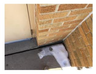
Photo 5. Caulk joint between building and exterior concrete. Water below slab could cause the slab to heave. (Priority 0)
