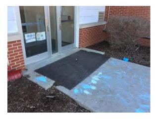
Photo 1. Exterior concrete sidewalk has separated from stoop slab. Sidewalk should be re-poured and tied into the stoop wall to avoid differential movement. (Priority 1).
