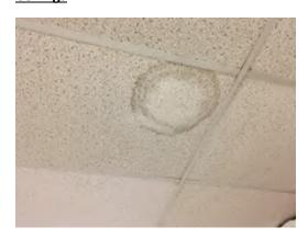
Photo 21. Water damaged ceiling tile from leak (origin unknown). ACT ceilings used in corridors and 2001 addition classrooms.
