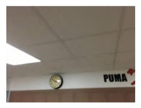
Photo 33. 2x2 Acoustical Ceiling Tile ceilings at  $1^{st}$  floor corridor of 1968 building. Ceiling in good condition.
