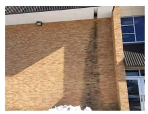
Photo 5. Brick discolored due to water run-off. Clean masonry. (Priority 0)
