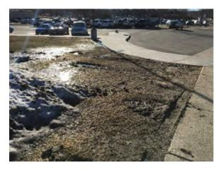
Photo 18. Rutting resulting from plowing operations. (Priority 0)
