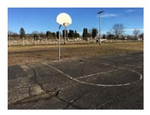
Photo 9. Asphalt in east play area in poor condition. This area should be patched or replaced. (Priority 3)
