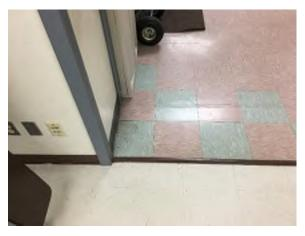
Photo 43. Cafeteria flooring (12x12 VCT) is cracking.
