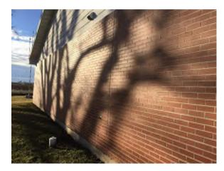
Photo 23. Masonry on 2000 addition in good condition. No visible signs of deterioration.
