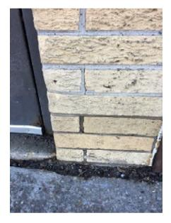
Photo 7. Brick throughout the 1954 exterior shows mortar cracking. Tuckpoint exterior. (Priority 0)
