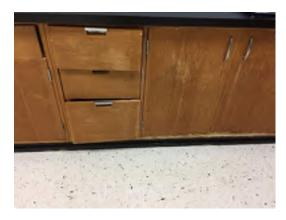
Photo 22. Casework in poor condition in 1963 classroom.
