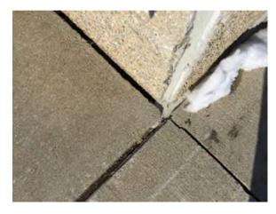
Photo 27. Joint between sidewalk and exterior wall should be reviewed and caulked as needed. Water infiltration below sidewalk slab could lead to heaving issues. (Priority 0)
