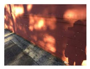
Photo 5. Paint peeling off exterior Gymnasium walls throughout. Remove existing and repaint. (Priority 0).
