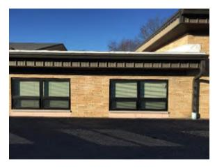
Photo 27. South elevation windows into 1954 classrooms were replaced and partially infilled in the last 10 years.
