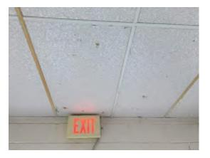
Photo 34. 2x4 ACT ceilings in 1954 building corridors. Tile and grid in poor condition. Tile should be replaced. (Priority 2)
