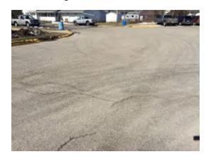
Photo 5. Miscellaneous asphalt cracking throughout. Chip seal and stripe. (Priority 0)  $\,$
