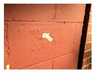
Photo 4. Paint peeling off exterior Gymnasium walls throughout. Remove existing and repaint. (Priority 0).
