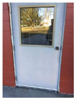
Photo 30. Exterior doors in poor condition. Need to be adjusted and sealed more effectively. (Priority 0).
