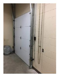
Photo 17. Automatic overhead door at 2012 addition. Door in good condition.
