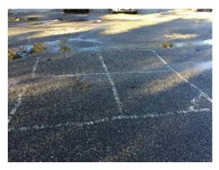
Photo 8. Asphalt in poor condition with cracking and potholes throughout. Replace and restripe. (Priority 0).
