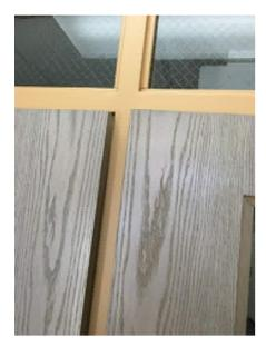
Photo 13. Doors at first floor vestibule in 1999 addition do not close. Check HVAC balancing to confirm pressurization. (Priority 1)
