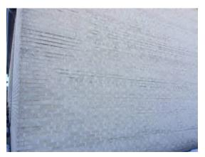
Photo 14. Brick at 1963 original building in good condition.
