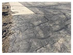
Photo 8. Asphalt in north play area in poor condition. This area should be patched or replaced. (Priority 3)
