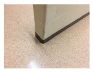
Photo 50. VCT flooring from 2012 building addition, in good condition.
