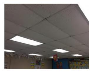
Photo 36. 2x4 ACT ceiling in 1989 addition classroom. Tile is sagging and in poor condition. To reduce issues with 2x4 tiles, retrofit to 2x2 grid and install 2x2 tile. (Priority 0)
