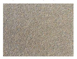
Photo 25. Texture of precast, typical 2001 addition.
