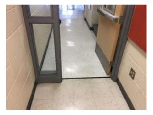
Photo 64. Flooring transition between two VCT products in corridor to the south of the gym.
