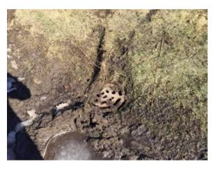
Photo 10. Landscaping around storm inlet to northeast of the main gymnasium should be cleared back to allow for proper drainage. (Priority 0)
