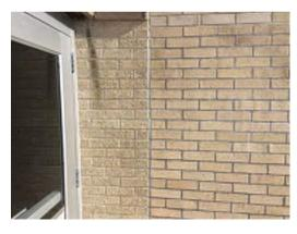
Photo 4. Brick to brick control joint on buildings south elevation
