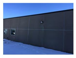
Photo 21. Precast panels installed at west wall of District Office, part of 2001 addition.
