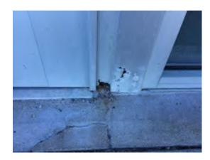
Photo 35. Aluminum door frame failing. These should be replaced. (Priority 2)
