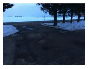
Photo 3. Asphalt in poor condition with cracking and potholes throughout. Replace and restripe. (Priority 0).
