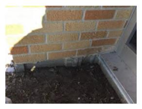
Photo 13. Concrete frost walls appear to come up to 8" below grade. One course of CMU is run around the exterior below brick. This is the 1968 Addition.
