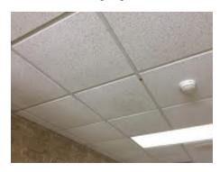
Photo 53. Water stained ceiling tiles are present throughout the N/S hallway on the east side of the gymnasiums. Flashing at roofline needs to be addressed.
