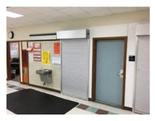
Photo 11. Wood trim and painted wood door into Kitchen from Cafeteria. Overhead roll-up doors also installed in multiple locations along south wall to kitchen. OH doors in good condition.
