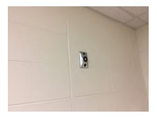
Photo 34. Magnetic hold opens are installed at areas in the 2001 addition.
