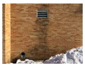
Photo 3. Brick discolored due to water run-off. Clean masonry. (Priority 0).
