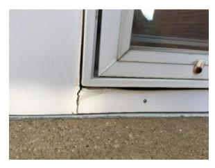
Photo 29. Exterior veneer failing at window on building's west elevation.
