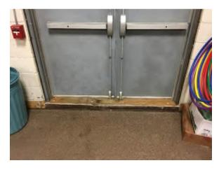
Photo 13. Exterior doors to north in poor condition. Daylight can also be seen at bottom. Replace or adjust, add weatherstripping.
