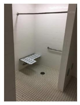
Photo 81. Shower unit is ADA accessible and has a bench and grab bars.
