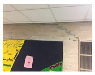
Photo 46. Brick wall finish in 1963 corridor has cracked and been repaired.
