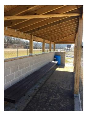
Photo 8. Southern softball field dugouts. CMU block and wood structure in good condition.
