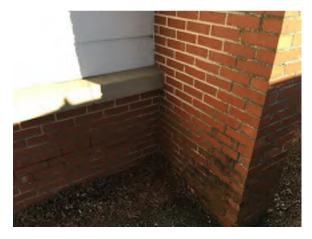
Photo 13. Mortar cracking and discoloration. Typical on west elevation.
