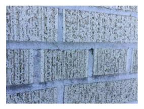
Photo 15. Brick at 1963 original building in good condition. Minor grout deterioration. Tuckpoint select areas. (Priority 0)
