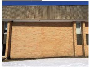
Photo 1. 1968 Exterior Wall, South Elevation. Brick in good condition.
