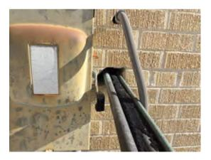
Photo 10. Caulk/seal openings on south elevation in brick. (Priority 0)
