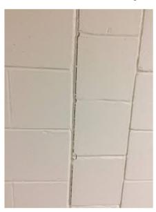
Photo 50. Crack in CMU wall at tie-in between 2001 addition (District Office Hallway) and 1963 original building. Install expansion control. (Priority 2)
