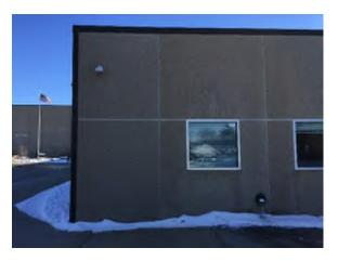
Photo 23. Crack is apparent in center of precast panel above window.
