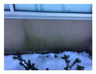
Photo 19. Moisture issue apparent at north elevation of 1963 classroom below window. Remove and replace failed backing material. (Priority 0)
