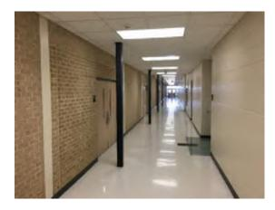
Photo 44. Exposed brick (1963 building exterior) on one side of the corridor with painted CMU in the 2001 addition.
