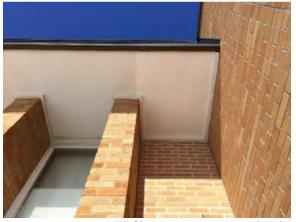
Photo 4. 1968 Exterior wall (left) at tie-in to 2012 addition (right). Soffit here in good condition, but mismatching colors.
