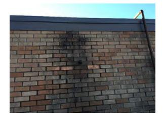
Photo 6. Brick discolored due to water run-off at 1954 original building. Clean masonry. (Priority 0)
