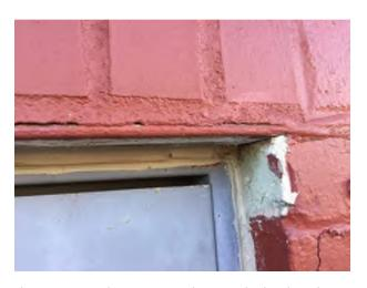
Photo 31. Exterior doors in poor condition. Need to be adjusted and sealed more effectively. Gap can be seen above as door in not square in frame.
