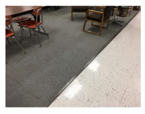
Photo 45. IMC carpeting and corridor 12x12 VCT. Flooring was replaced as part of the 2012 work. Good condition.
