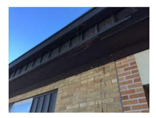
Photo 18. Tie-in of 1999 addition (right) to original 1954 building (left). Prep and repaint original 1954 soffit boards. (Priority 2)
