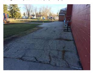
Photo 7. Asphalt in poor condition with cracking and potholes throughout. Replace and restripe. (Priority 0).
