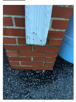
Photo 13. Asphalt has failed and roof runoff runs between asphalt and the building. Install corrective measure to direct water away from the building.
