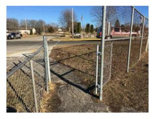
Photo 15. Gate along NE boundary of site. Play area not fully enclosed or secure. Include gates at openings to close off play area. (Priority 2)
