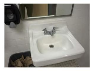
Photo 78. Manual valve faucets are installed in the 2001 addition bathroom.
