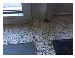
Photo 30. Aluminum frame is rusting at the intersection with the floor. (Priority 2).
