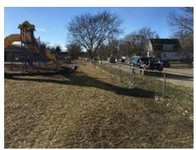
Photo 14. Fencing along north boundary of site is bent and damaged. Fencing should be replaced with a taller fence along E. Seward Street. (Priority 2)
