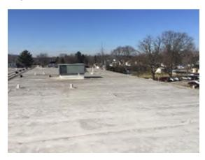
Photo 39. Roofing at 1963 original building. Roofing rework was completed in 2014.
