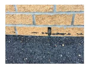
Photo 12. Weep vent at 1989 addition north elevation is plugged. Review weep vents throughout to confirm proper drainage out of wall cavity. (Priority 0)
