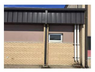
Photo 7. Downspouts on south side of building discharge at grade on a sphalt paving.  $\label{eq:controller}$
