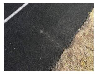
Photo 6. Cracking along the outside edge of the running track.
