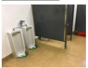
Photo 55. Manual flush valve urinals in 1954 building. Toilet partitions have been replaced and are in good condition.
