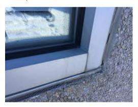
Photo 34. Caulk joint is failing a 2001 window in precast. (Priority 0)
