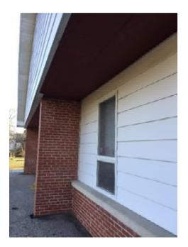
Photo 9. East side exterior wall and painted wood soffit.
