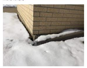
Photo 12. Brick overhangs foundation wall slightly on south elevation.
