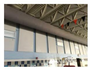
Photo 47. Painted block walls in the pool area. Acoustical wall panels installed throughout.
