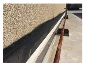
Photo 40. Roofing tie-in at south wall of 2001 gymnasium. Address flashing detail, water infiltration is a consistent issue here. (Priority 0)
