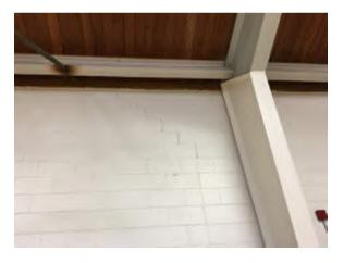
Photo 25. Masonry walls at gymnasium. Cracking is seen throughout the south wall. Route and caulk. (Priority 0)
