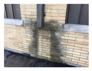
Photo 10. Brick discolored due to water run-off at 1954 original building. Clean masonry. (Priority 0)
