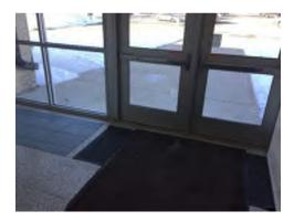
Photo 59. Walk-off mats installed over terrazzo at building entry on north elevation.
