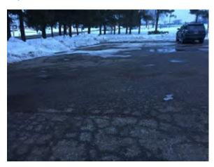
Photo 2. Asphalt in poor condition with cracking and potholes throughout. Replace and restripe. (Priority 0).
