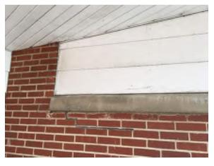
Photo 16. Masonry cracking at main entrance.
