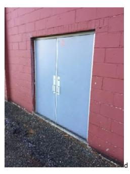
Photo 28. Gymnasium exterior doors, facing north. Doors need to be adjusted, and additional weatherstripping installed. Large gap at bottom of door. (Priority 0).
