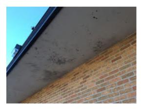
Photo 15. Soffit of 1989 addition shows discoloration. No venting mechanism is apparent. Remove soffit panels and investigate discoloration. Replace soffit as necessary and cut in venting to allow air transfer. (Priority 0)
