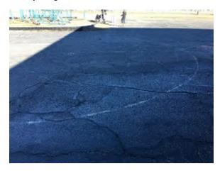
Photo 11. Asphalt in east play area in poor condition. This area should be patched or replaced. (Priority 3)
