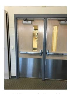
Photo 38. Music rooms with hollow metal framing and wood door hardware. Panic bars installed in the door for means of egress.
