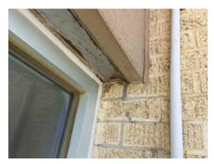
Photo 18. Typical window on 1963 building north elevation. Lintel is unpainted, finish of wall system in fair condition. (Priority 3)
