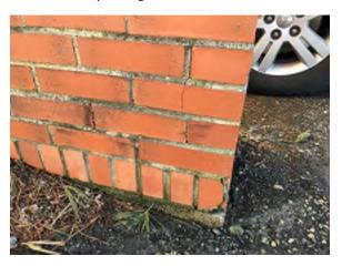
Photo 17. Masonry cracking at main entrance.
