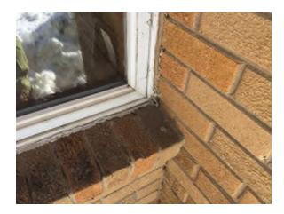
Photo 32. Caulking failed at 1989 addition windows. Cut out and replace. (Priority 0)
