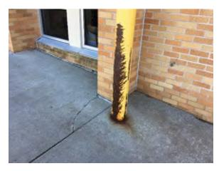
Photo 4. Paint should be reapplied at exterior bollard, northwest portion of the site.
