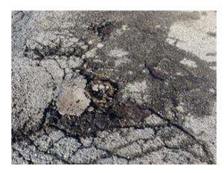
Photo 6. Asphalt in poor condition with cracking and potholes throughout. Replace and restripe. (Priority 0).
