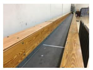
Photo 95. Bleachers in Auxiliary Gym should be replaced at end of useful life. (Priority 2)
