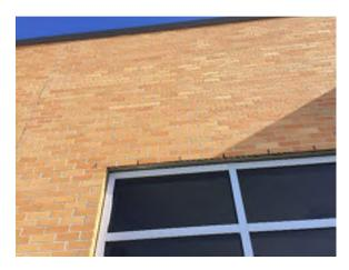
Photo 23. Lintels are primed steel and show signs of rust. Paint exterior lintels at 2012 addition.
