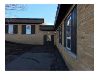
Photo 20. Address drainage in nook along north elevation of 1954 original building.
