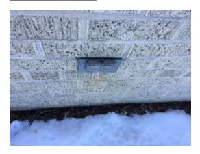
Photo 1. Receptacle on exterior wall. Visible gap between brick.
