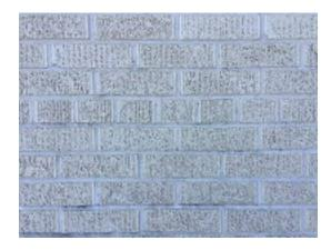
Photo 13. Brick at 1963 original building in good condition.
