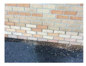
Photo 11. The surface of the brick at the north elevation of the 1968 addition is deteriorating. It appears that snow may be plowed against this wall in the winter. This should be avoided to maintain integrity of brick.
