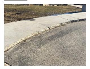
Photo 1. Curb is damaged at southeast section of the site.
