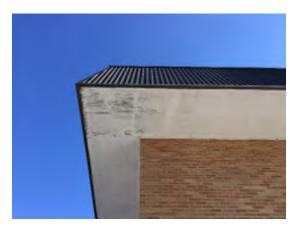
Photo 14. Soffit of 1989 addition shows discoloration. No venting mechanism is apparent. Remove soffit panels and investigate discoloration. Replace soffit as necessary and cut in venting to allow air transfer. (Priority 0)
