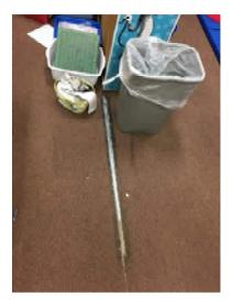
Photo 24. Carpet seam pulling apart. Carpet is very worn and in poor condition. Yearly allowance is included for finish repair/replacement throughout the building.
