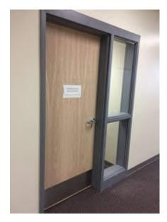
Photo 36. Hollow metal frame with sidelite and wood door at the 2001 District Office addition. Lever handle with keyed access.
