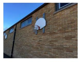
Photo 26. 1954 building north elevation. Basketball station mounted directly to exterior wall.
