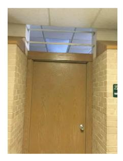
Photo 32. Area above doors open between hallway and classrooms in 1963 original building utilized for air flow. Solution not addressed as part of the assessment.
