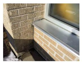
Photo 2. Detail at window and adjacent wall on building south elevation. Review caulking and sealing when differing materials intersect. (Priority 0)
