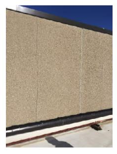
Photo 41. South elevation of 2001 gymnasium addition, on roof. Vertical cracking is present at middle of each panel. Cracks should be monitored and recaulked as needed. (Priority 0)
