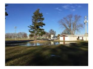
Photo 14. Site drainage issues at NE corner of site. Standing water present. Fill and regrade to improve drainage. (Priority 0).
