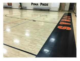
Photo 97. Gym flooring in Auxiliary Gym in good condition. Floors are maintained yearly.
