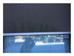
Photo 20. Moisture issue apparent at north elevation of 1963 classroom window head. Remove and replace failed backing material. (Priority 0)
