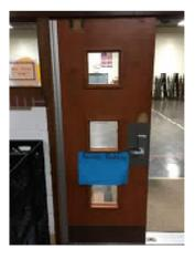
Photo 12. One leaf of doors from entrance hallway into gymnasium. Door hardware retrofitted and leaves stain mismatched.
