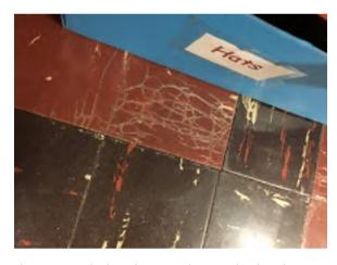
Photo 25. 9x9 Tile Throughout is cracking at isolated conditions and in poor condition.
