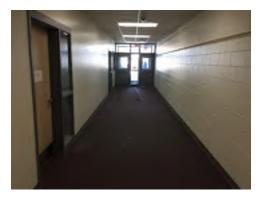
Photo 60. Carpeting installed in the main District Office hallway. Carpet in good condition. Walk off mats installed adjacent the vestibule.
