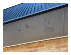
Photo 17. Soffit paint finish on exterior peeling away, prep and repaint. Venting may need to be added similar to other areas. (Priority 0)
