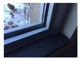
Photo 17. Solid surface window sills at north elevation of 1963 original classrooms are in good condition.
