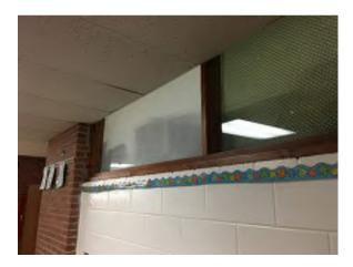
Photo 5. Clerestory glazing from classrooms to corridor. Ceiling returns to accommodate as much light to enter corridor as possible.
