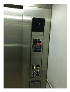
Photo 77. Elevator services floors 1 and 2 of the building and was installed in the 2001 addition. Elevator is inspected regularly.
