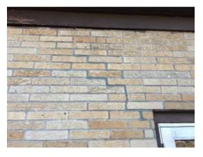
Photo 9. Brick throughout the 1954 exterior shows mortar cracking. This location has been caulked.
