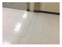
Photo 58. Vinyl flooring crack at the  $2^{nd}$  floor between 1963 original building and 2001 addition. Install expansion to address movement issues. (Priority 2)
