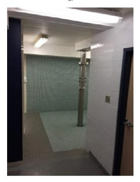
Photo 65. Multiple flooring tile colors are installed in the shower area of the boys locker room.
