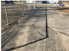
Photo 6. Asphalt in north play area in poor condition. This area should be patched or replaced. (Priority 3)
