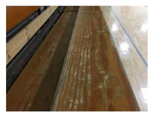
Photo 96. Bleachers in Auxiliary Gym should be replaced at end of useful life. (Priority 2)
