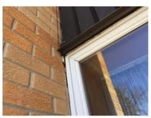
Photo 31. Caulking failed at 1989 addition windows. Cut out and replace. (Priority 0)
