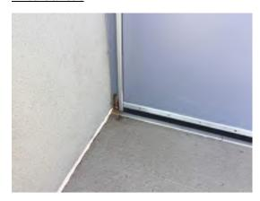
Photo 29. Bottom of hollow metal door frame is shows signs of deterioration. Replace or repair frame. (Priority 1)
