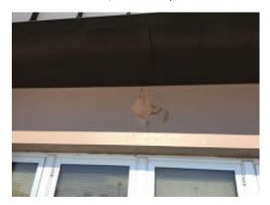
Photo 9. Finish delaminating in an isolated location on the south elevation. Repair finish. (Priority 0)
