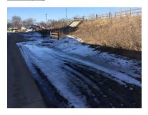
Photo 7. Rutting present around gymnasium from plowing operations.
