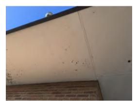
Photo 16. Soffit of 1989 addition shows discoloration. No venting mechanism is apparent. Remove soffit panels and investigate discoloration. Replace soffit as necessary and cut in venting to allow air transfer. (Priority 0)
