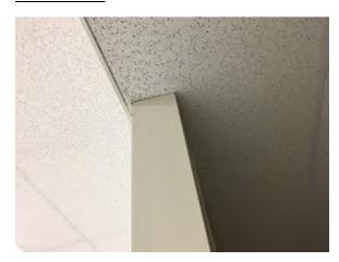
Photo 20. Drywall partition walls installed after ceiling in perimeter classrooms around IMC.
