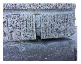
Photo 16. Brick at 1963 original building in good condition. Minor grout deterioration. Tuckpoint select areas. (Priority 0)
