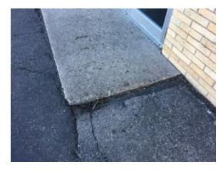
Photo 3. Differential movement at exterior concrete slabs. This should be replaced or remedied. (Priority 2)
