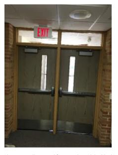
Photo 12. Hollow metal frame and wood double doors in 1999 addition.
