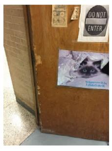
Photo 25. Door to maintenance area in main 1963 corridor. Replace door on first floor. (Yearly finish allowance included in Capital Maintenance Planning Budgets – Section 09)
