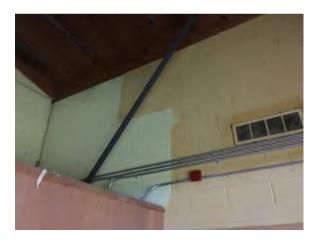
Photo 22. Finishes at stage in 1954 original building inconsistent.
