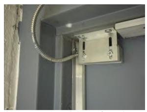
Photo 26. Door monitoring in place to assess if exterior doors are left open.
