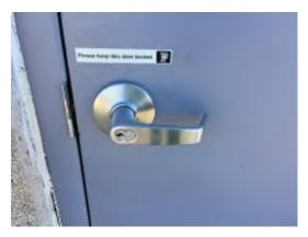
Photo 36. Keyed lever handle on 2001 building exterior.
