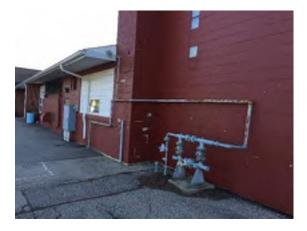
Photo 15. Gas meter exposed adjacent hard play area. Screen gas meter to separate from students. (Priority 0).
