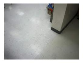
Photo 56. 9x9 vinyl flooring tiles installed at various classrooms in 1963 building. 9x9 tile is indicative of asbestos containing flooring/mastic.
