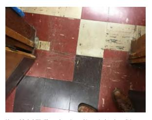
Photo 26.  $9\mathrm{x}9$  Tile Throughout is cracking at isolated conditions and in poor condition.
