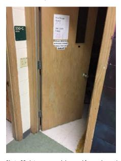
Photo 33. Art room wood door and frame shows signs of wear, in fair condition. Knob door hardware.
