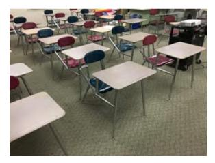
Photo 73. Carpet at second floor 2001 addition classroom is fair condition. Showing signs of wear, staining.
