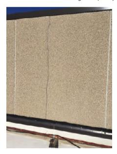
Photo 28. South elevation of 2001 gymnasium addition, on roof. Vertical cracking is present at middle of each panel. Cracks should be monitored and recaulked as needed. (Priority 0)
