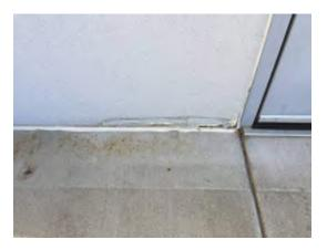
Photo 11. Finish damage at north aluminum entrance. Repair finish (Priority 0)
