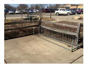
Photo 11. One set of loose bicycle racks at HS entry. Metal bars are bent throughout.
